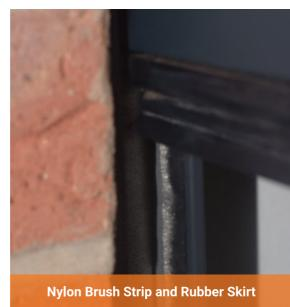
Installed to the bottom of your garage door is a durable rubber seal that helps to keep dust and debris from entering your garage.
